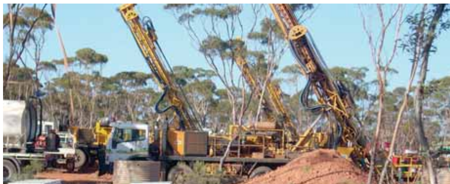
St Ives – Resource definition drilling at the Athena Project
