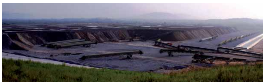
North Heap Leach phase V expansion
