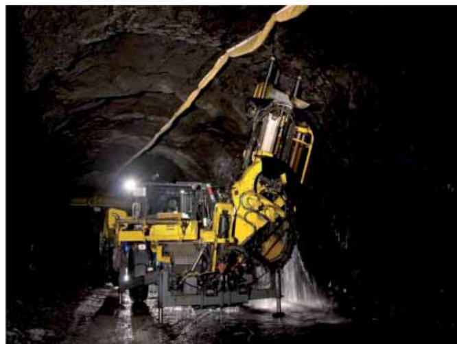
Simba drill rig – drilling longhole stope 95 1West
