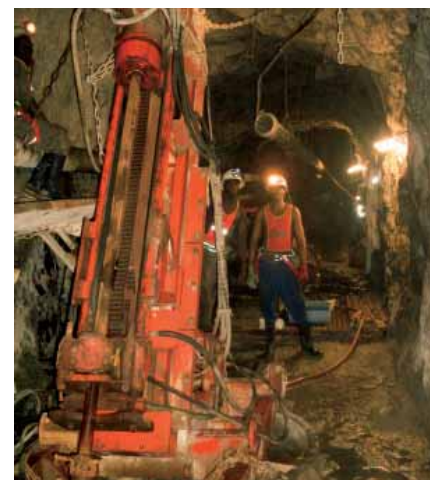
Underground Roco drilling machine capable of drilling boreholes in excess of 1,000 metres in length
