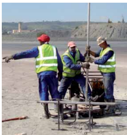
Tailings drilling activities
