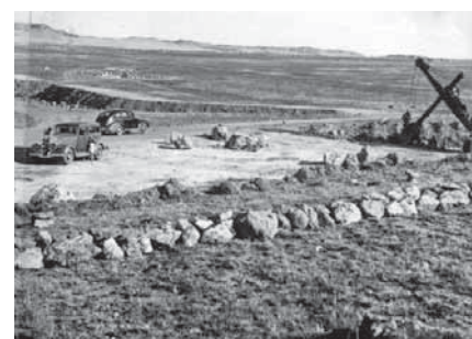
Driefontein 2 Shaft ground works, 16 September 1945
