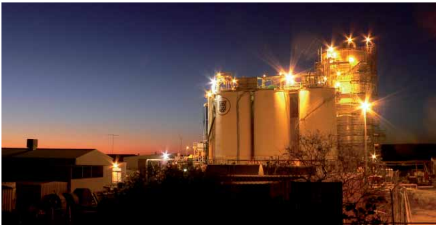
CIP processing plant
