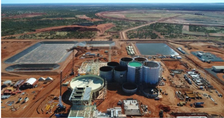
Gruyere plant, TSF and stage 1 pit
