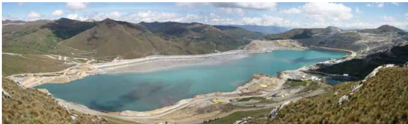
The Las Tomas reservoir at Cerro Corona, Peru
