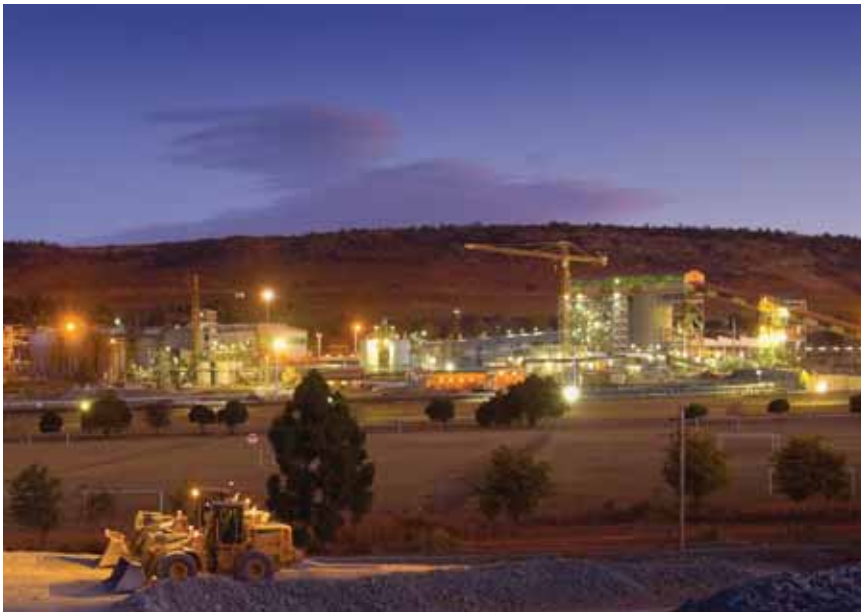
Surface operations at KDC East, South Africa
